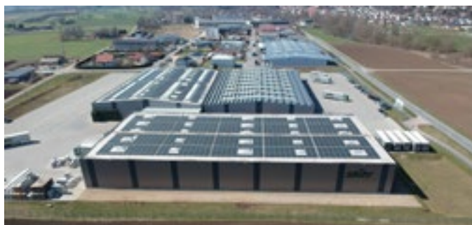
Stöhr Logistik | Rottenacker 544 kWp | SolarEdge Technik
